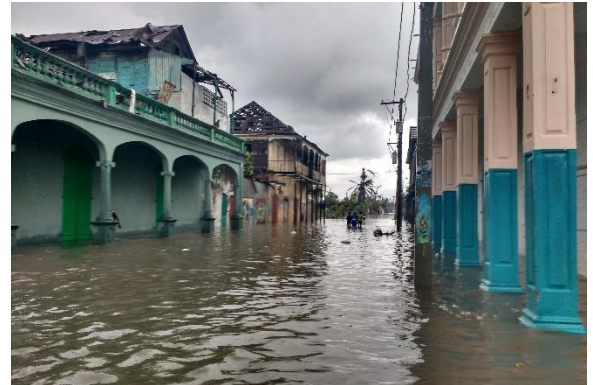
Recent heavy rainfall caused additional flooding in areas of southwestern Haiti already suffering due to Hurricane Matthew.
